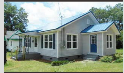
AFTER CONSTRUCTION PHOTO
