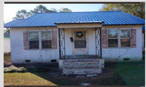
BEFORE CONSTRUCTION PHOTO
